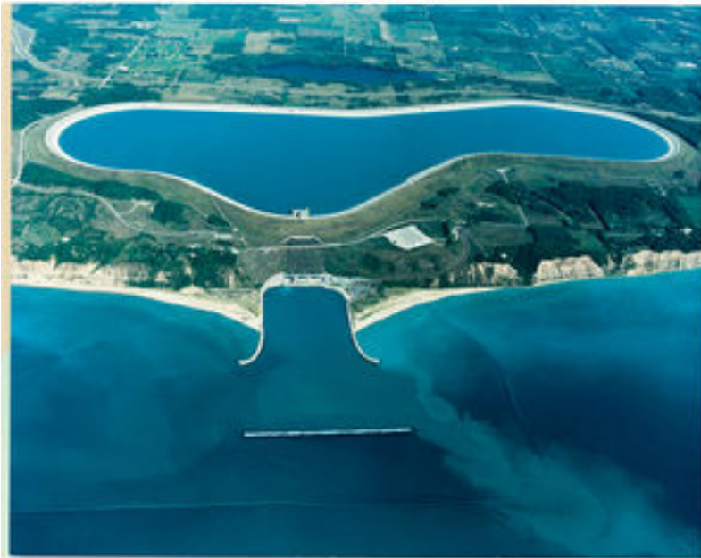
Ludington Pumped Storage Plant, Ludington, MI
